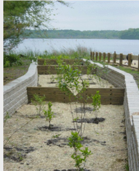
Vegetated swale at Long Lake
