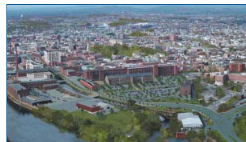
View of new Canal Street Bridge and Gateway site – prepared for the Gateway Task Force.
