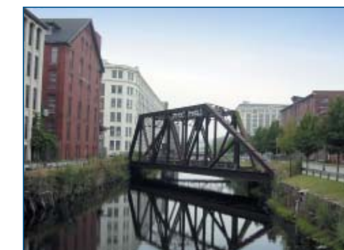
Canal bridges contribute to the area's unique identity.
